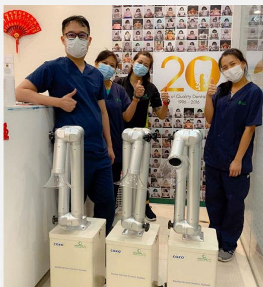
Photo of aerosol suction machines installed in clinics
